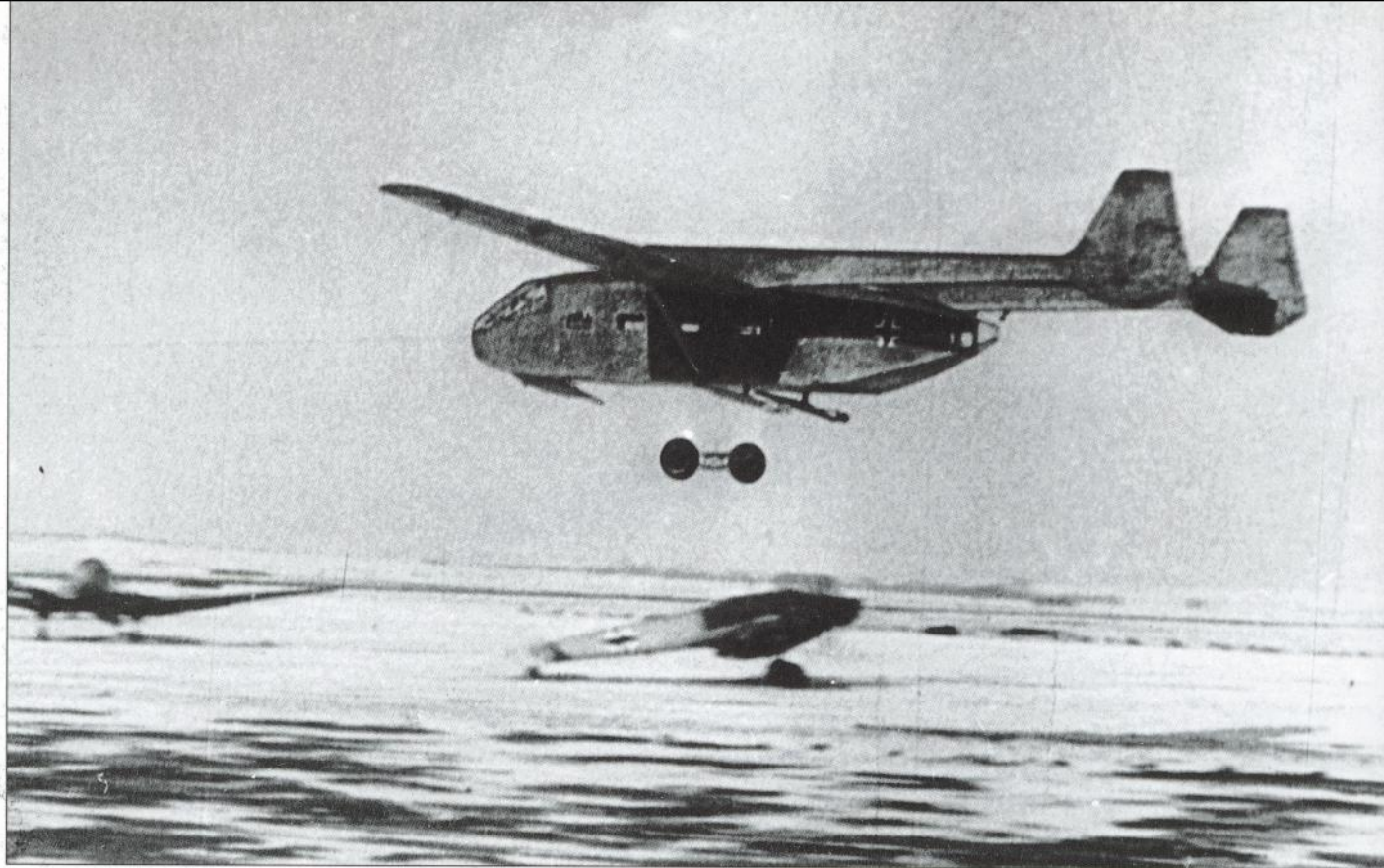
Above: A Gotha Go 242A assault and transport glider lifts off under tow, winter 1943-44. The aircraft is dropping its wheels to make it lighter and to improve aerodynamic shape.
