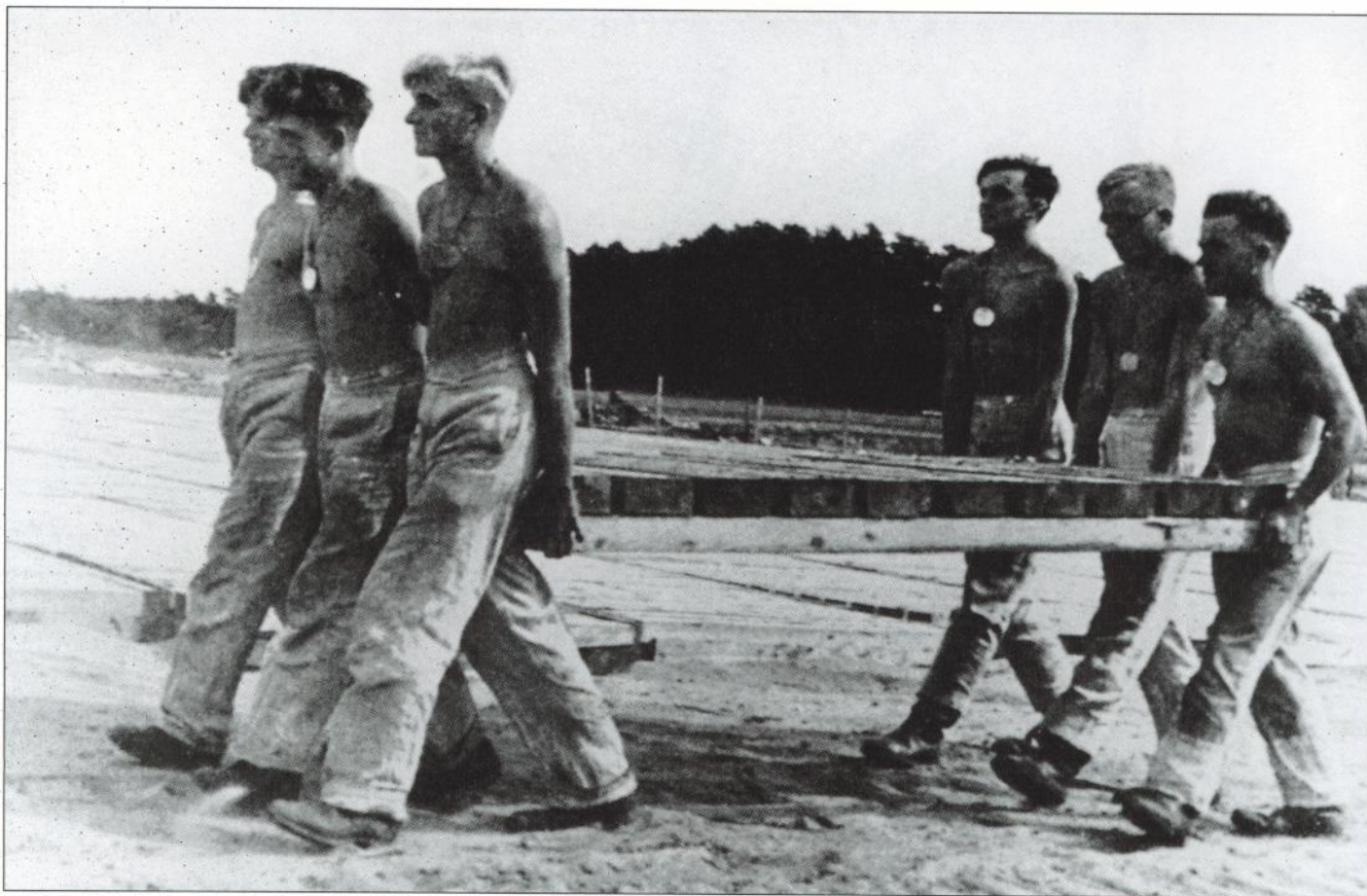
Above: Men of the Reichsarbeitsdienst (RAD), or State Labour Service, help to repair and extend the captured airfield at Oslo-Fornebu, April 1940. Here, they are carrying wooden segments of planking that will be employed to extend the runway, enabling it to be used by twin-engined Bf 110s.
